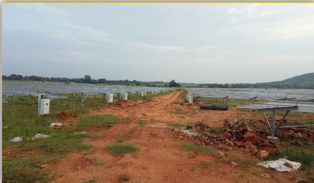
Figure 3: Internal Road access
