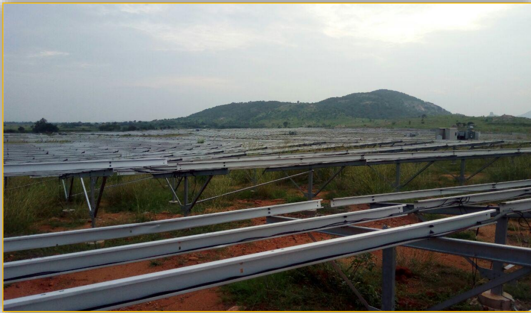
Figure 2 : MMS structure erected at OG Kuppam project site
