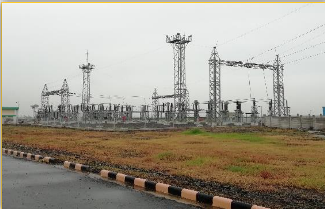
Figure 4: 132 kV Switchyard
