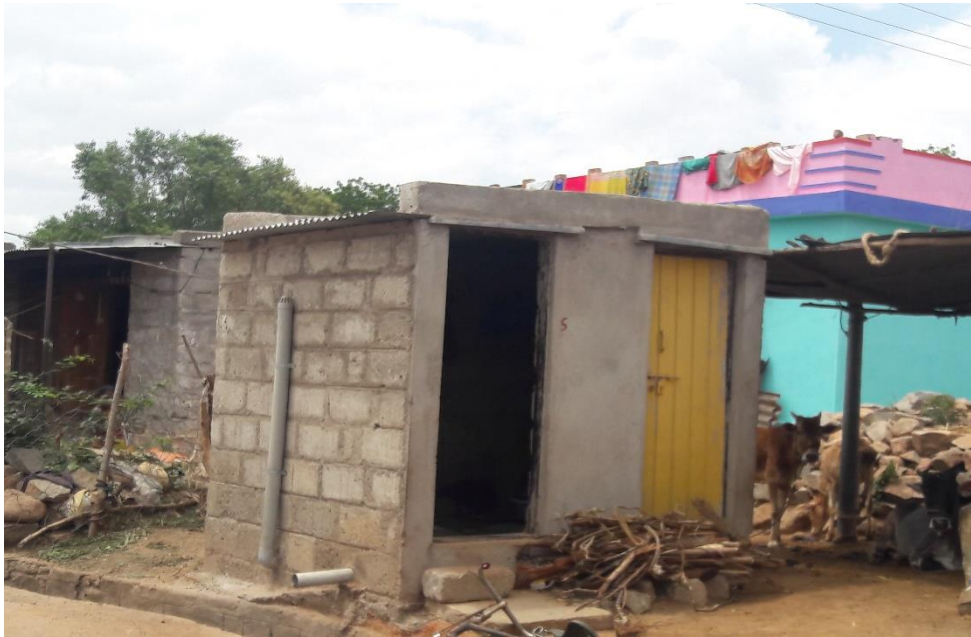
Pic 4-12 : Toilet Facility at Study area Village
