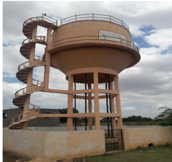
Pic 4-11: Water Tank at Village near the project site
