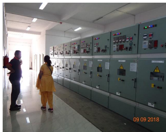
Visit to Project Site
