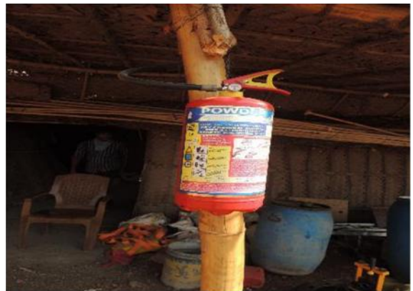
Photo 6-8: Fire extinguishers placed at camp
