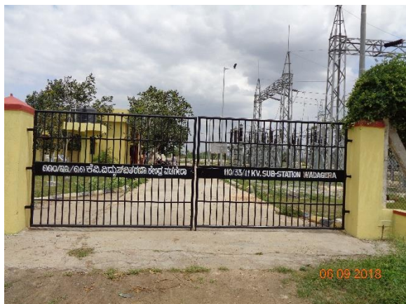
Pic 4-11: Sub station near the wadgera village
