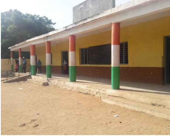
Pic 4-3: Primary school at Wadgera
