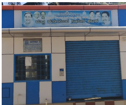
RO Water Filtration Plant at Kasapura village
