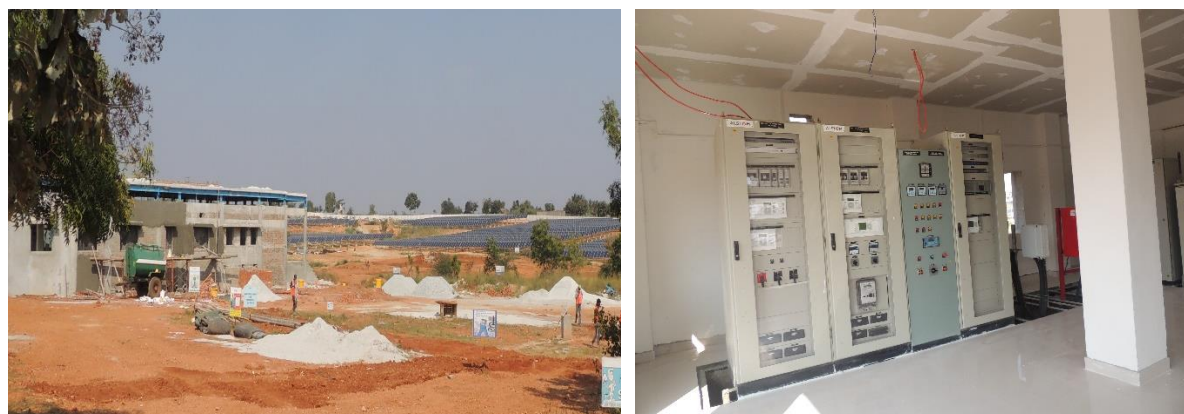
Figure 2-1: Construction Work at the Site
