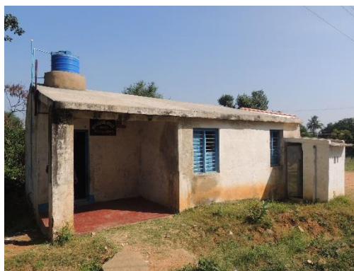
Roof Top tank at the ICDS centre in Kasapura
