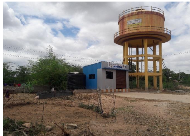
Figure 4-19: Tank as a source of water for the site area
