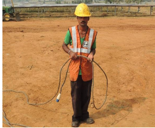
Laborer with PPE at Project Site
