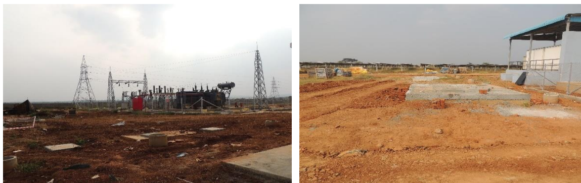
Figure 2-1: Construction Activities at the Site
