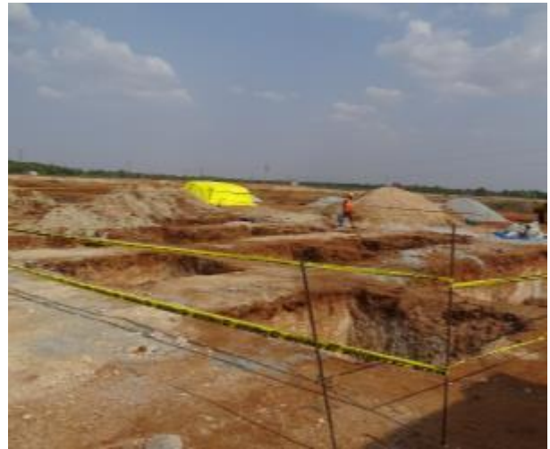
Photo 2-2:Commencement of construction works at site
