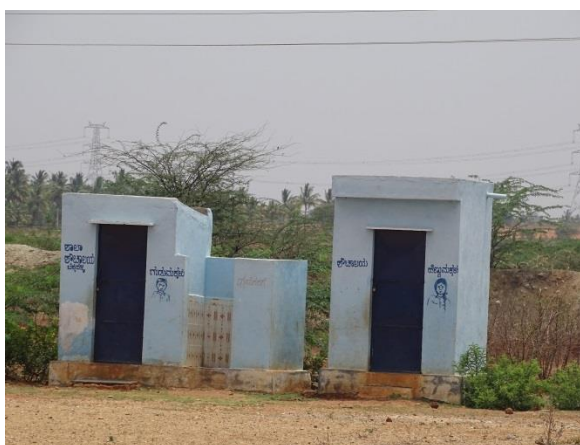
Photo 4-5: Sanitation facility in the village school
