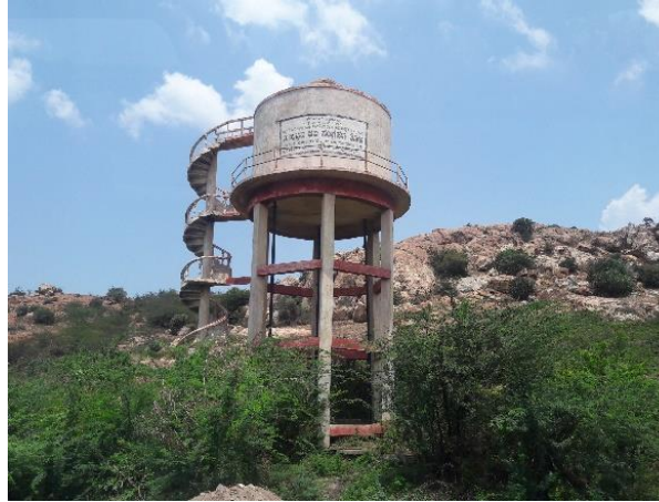
Pic 4-8 : Over head water Tank at K. Veerapura
