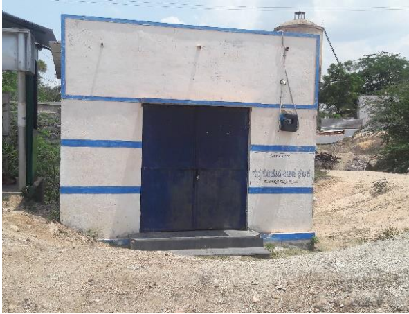
Pic 4-7 : RO Plant at K. Veerapura
